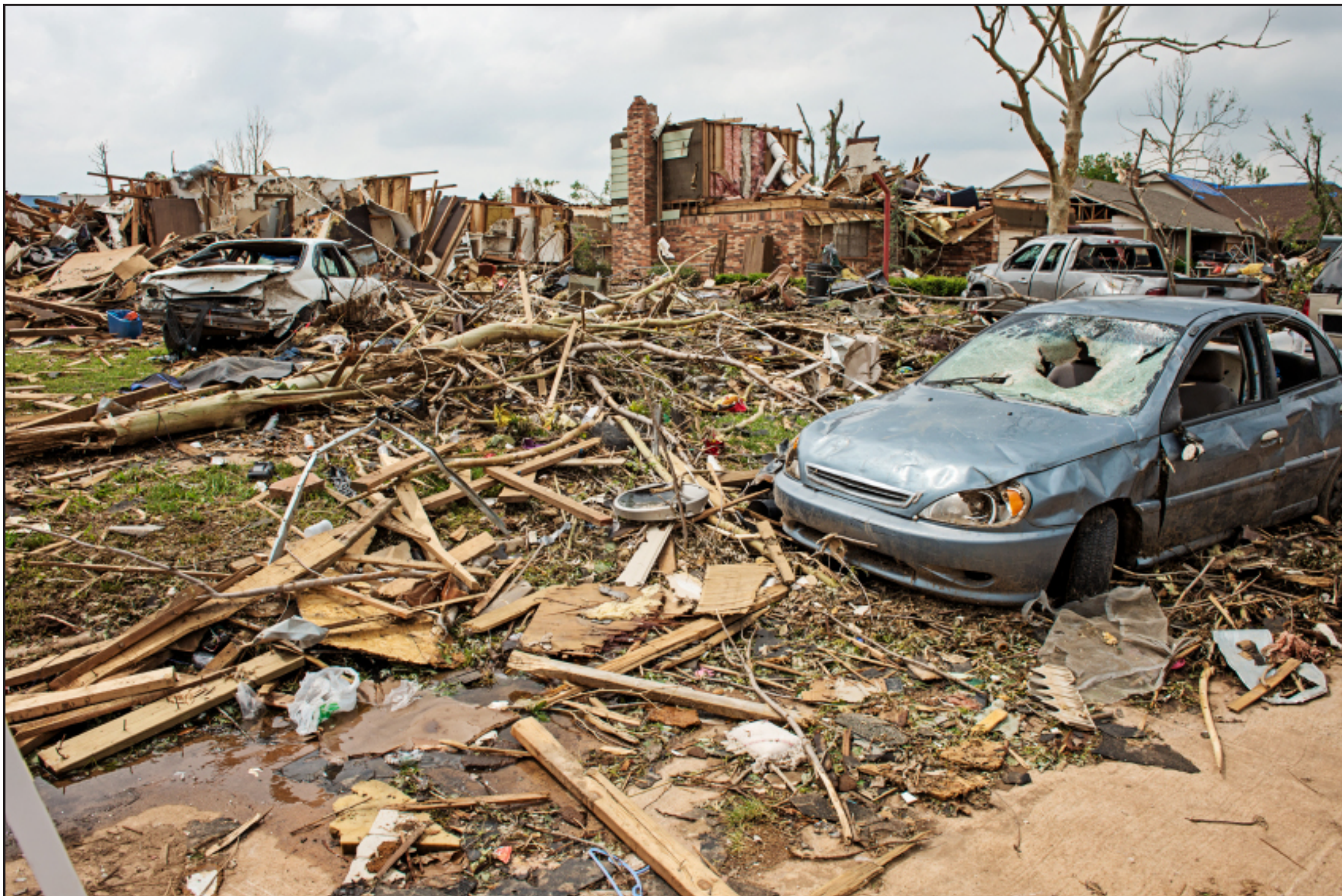
Destruction after a tornado in Oklahoma, USA on May 20th 2013.
