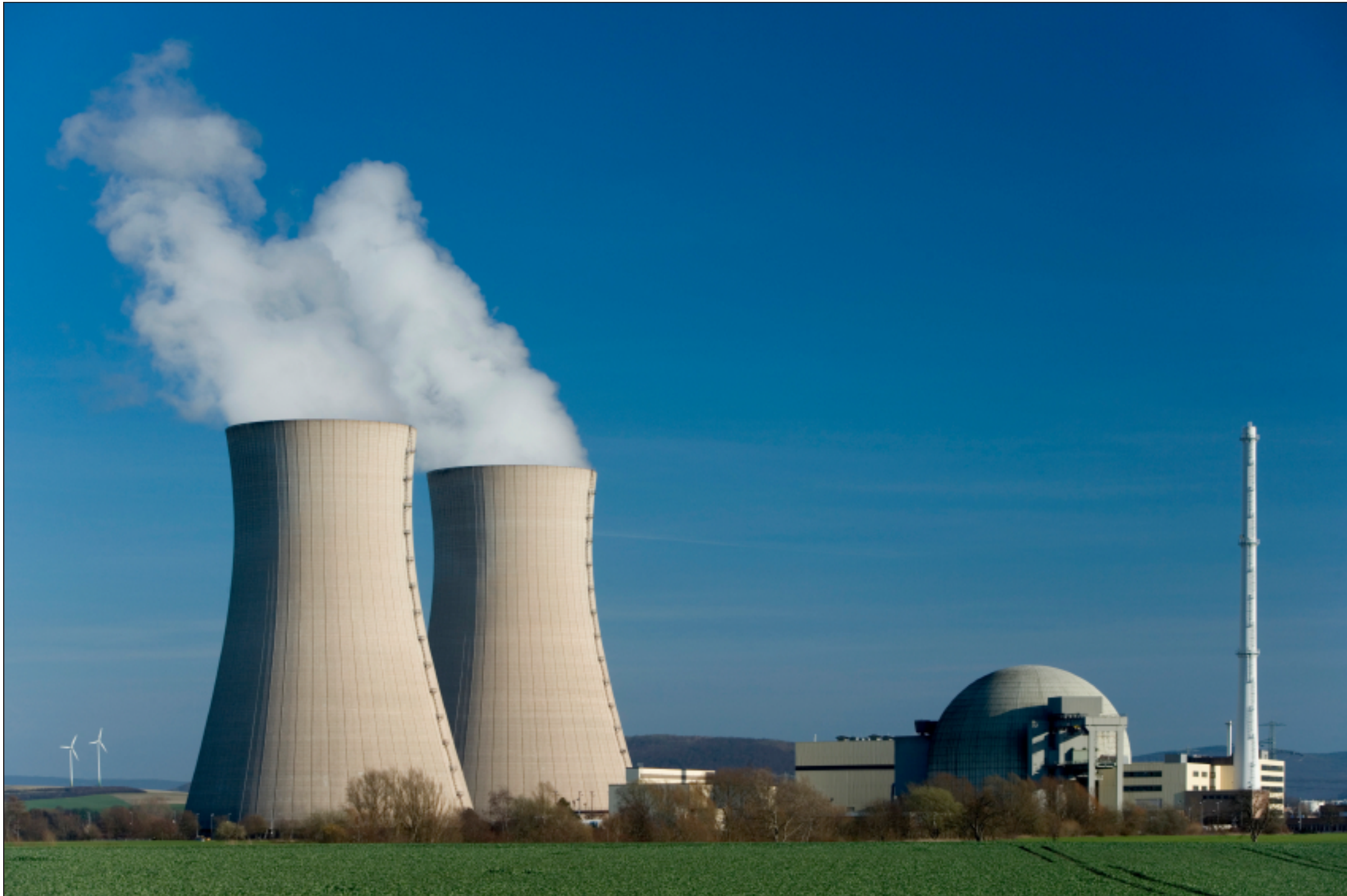
Grohnde, a nuclear power plant in Germany.
